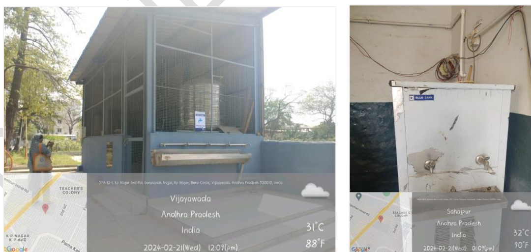
Plate 12: RO plant and water cooler facility in the premises
