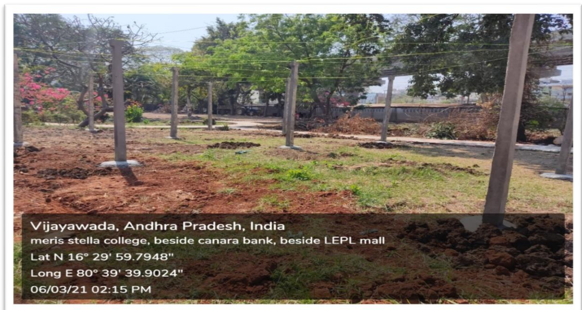
Construction of shade net in the campus on 06.03.2021
