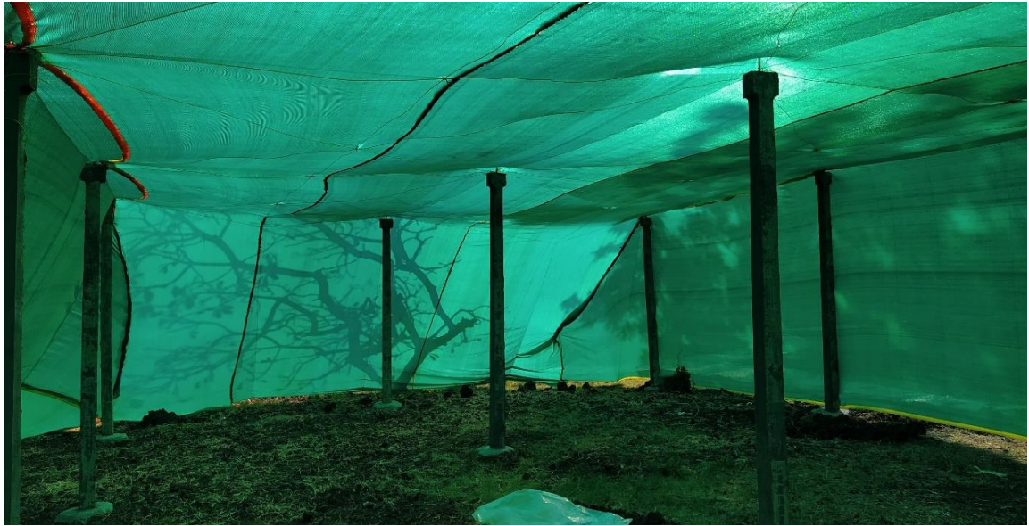
Completed shade net structure
