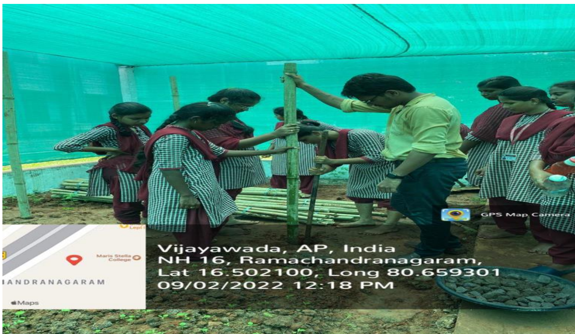
Construction of vertical garden in the polyhouse
