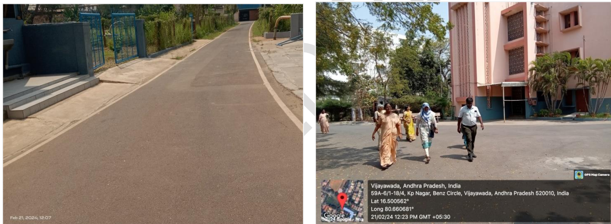
Plate 6: Wide roadways inside the premises
