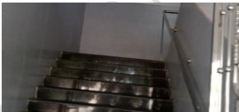
Plate 10: Staircase with handrail
