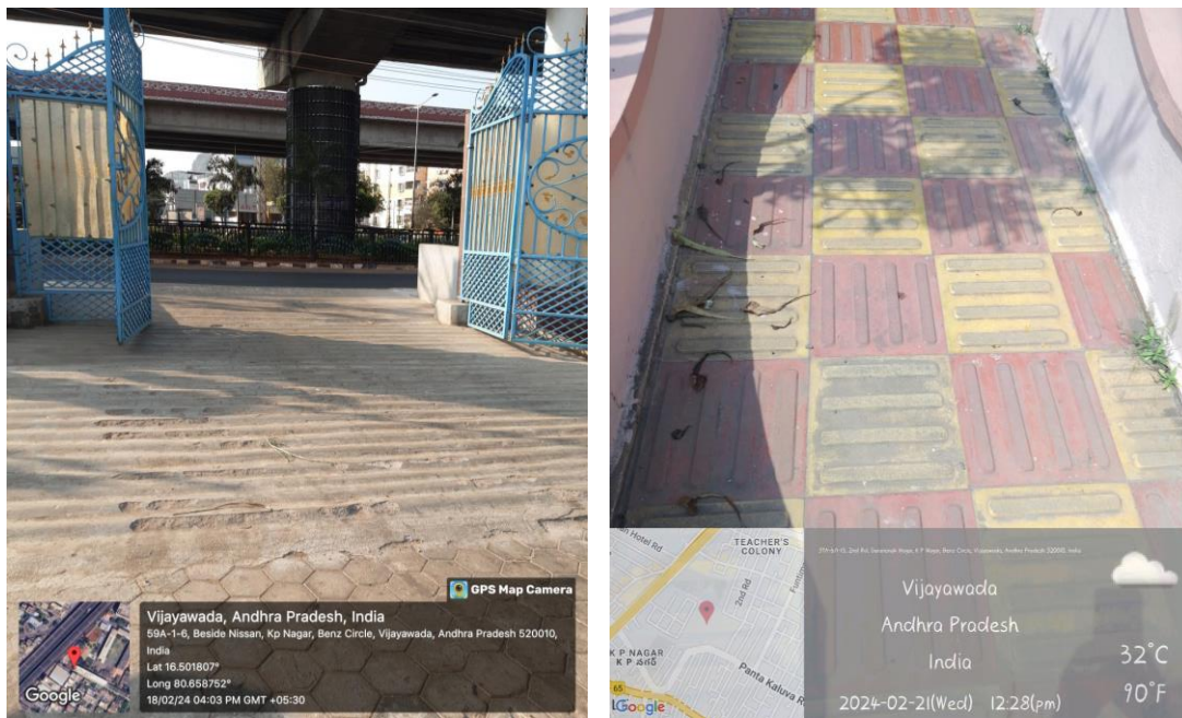
Plate 5: Non-slippery flooring material used at the main entrance and inside the premises
