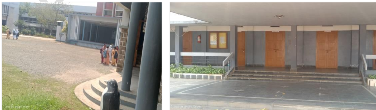
Plate 7: Wide access with steps made of non-slippery materials, handrail as and when required
